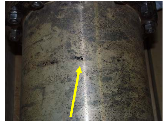
Water weep holes in transformer section
